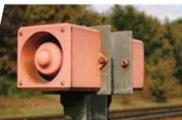
Example of a TOWS warning siren
